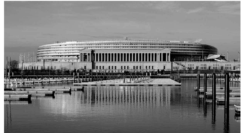
Soldier Field Renovation. Architects: Lohan, Caprile & Goettsch and Wood + Zapata. Photographed by David Seide ( www.DefinedSpace.com ).
